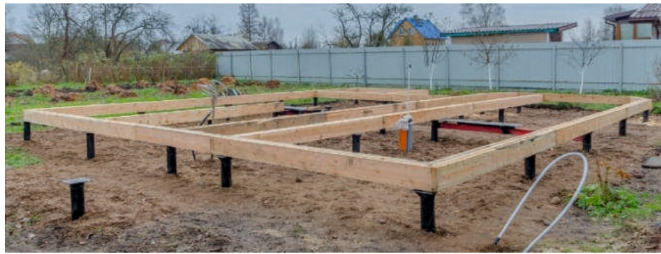
Timber subframe on ground screws.
