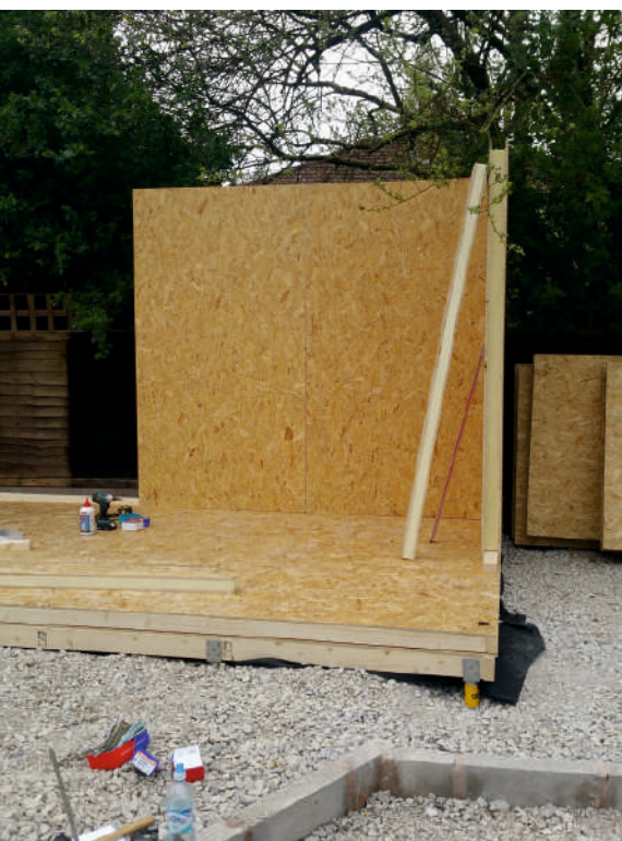
Constructions of wall started from a corner.
