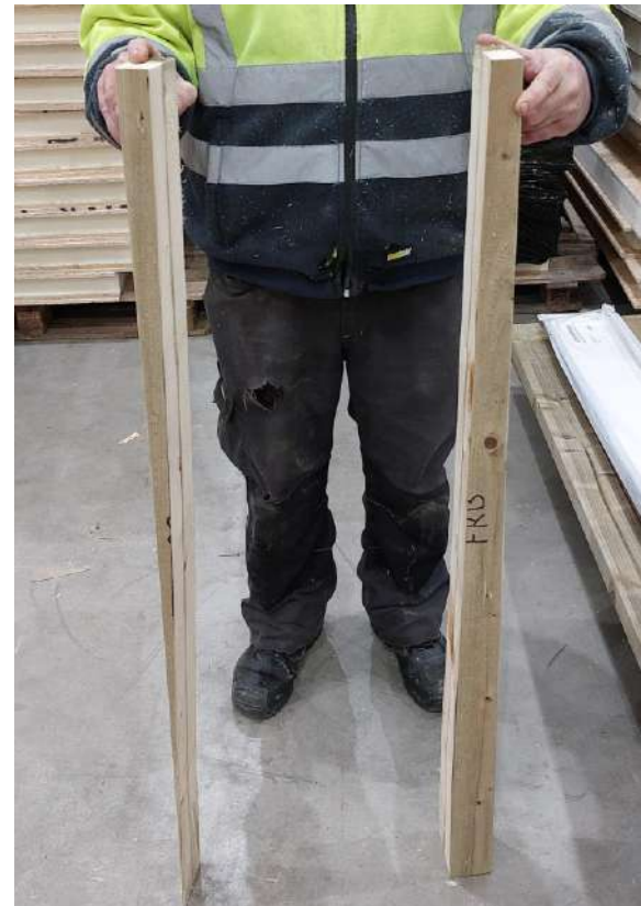
The firrings will usually come in two halves stacked on top of the other. Simply fix these next to each other.
