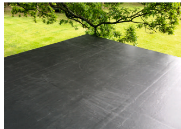
EPDM rubber roof installed.
