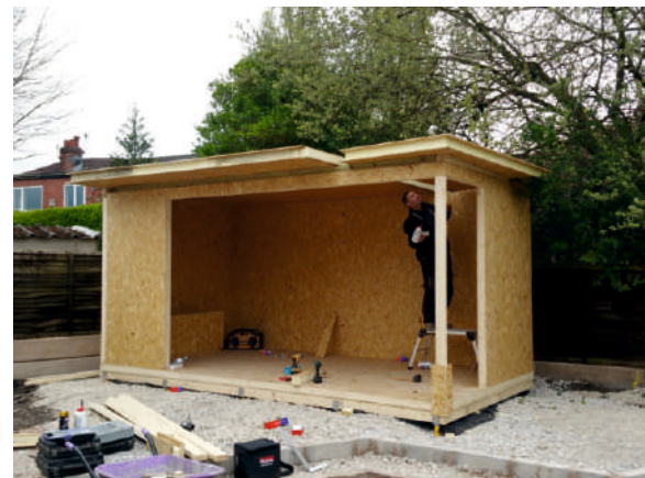
SIP roof being finished.
