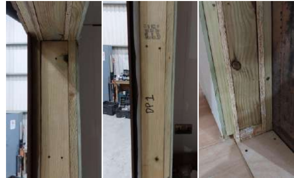
Finished door & window openings.
