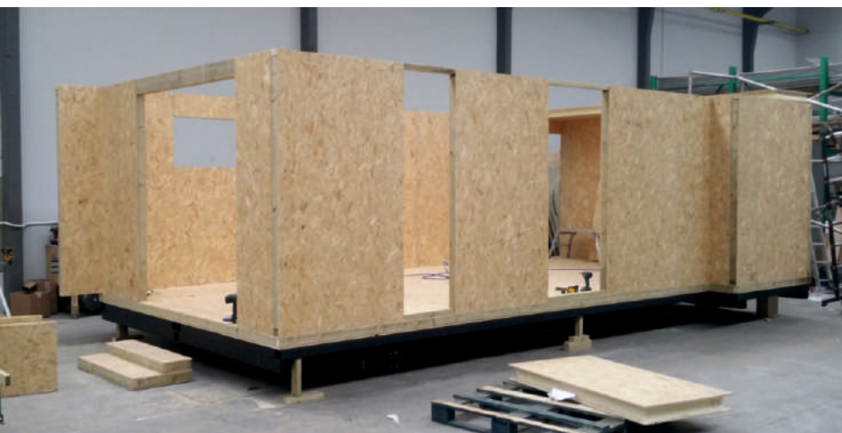
SIPs built to shell on a chassis.
