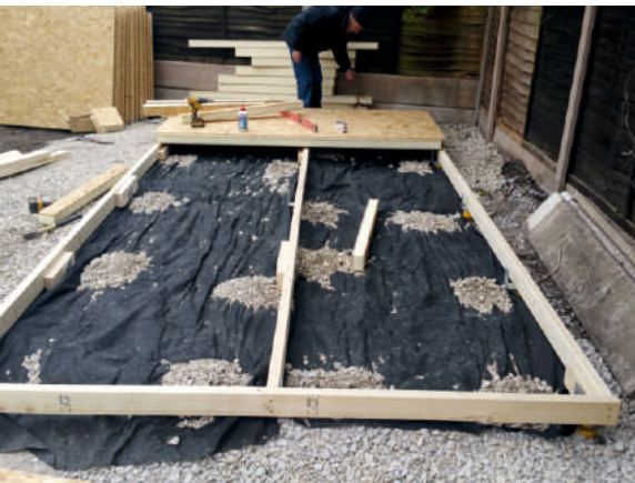
Floor SIP being attached to a timber subframe.
