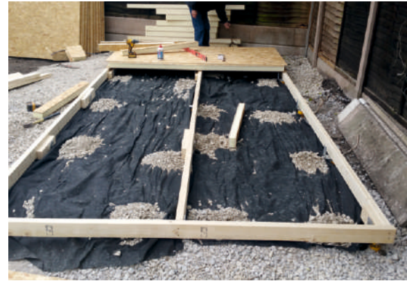
Photo: Example of a timber subframe with a SIP Floor Panel being installed.
